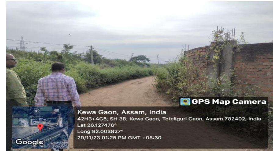
Photo Plate 6- Boundary wall need to demolish during the widening of the road. (Ch. 75.00 mts)
